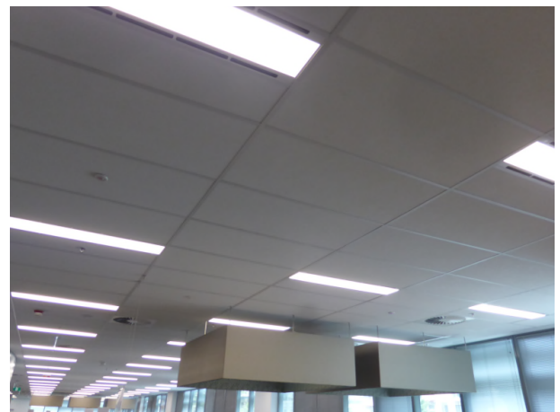
Figure 10: Photo showing regular grid
