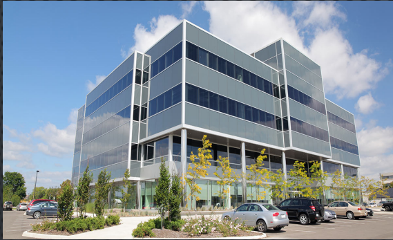
Whole Complex Chilled Water System
